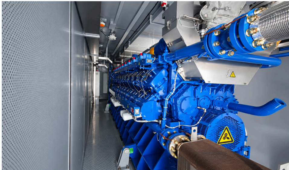
Internal view: engine, alternator and service access
